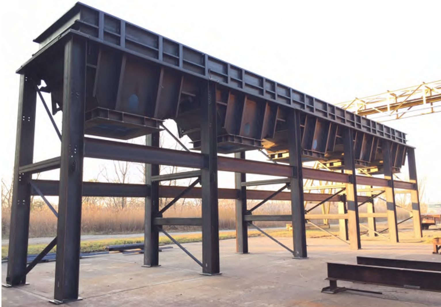
UCC PAX Hopper Trial Erection
