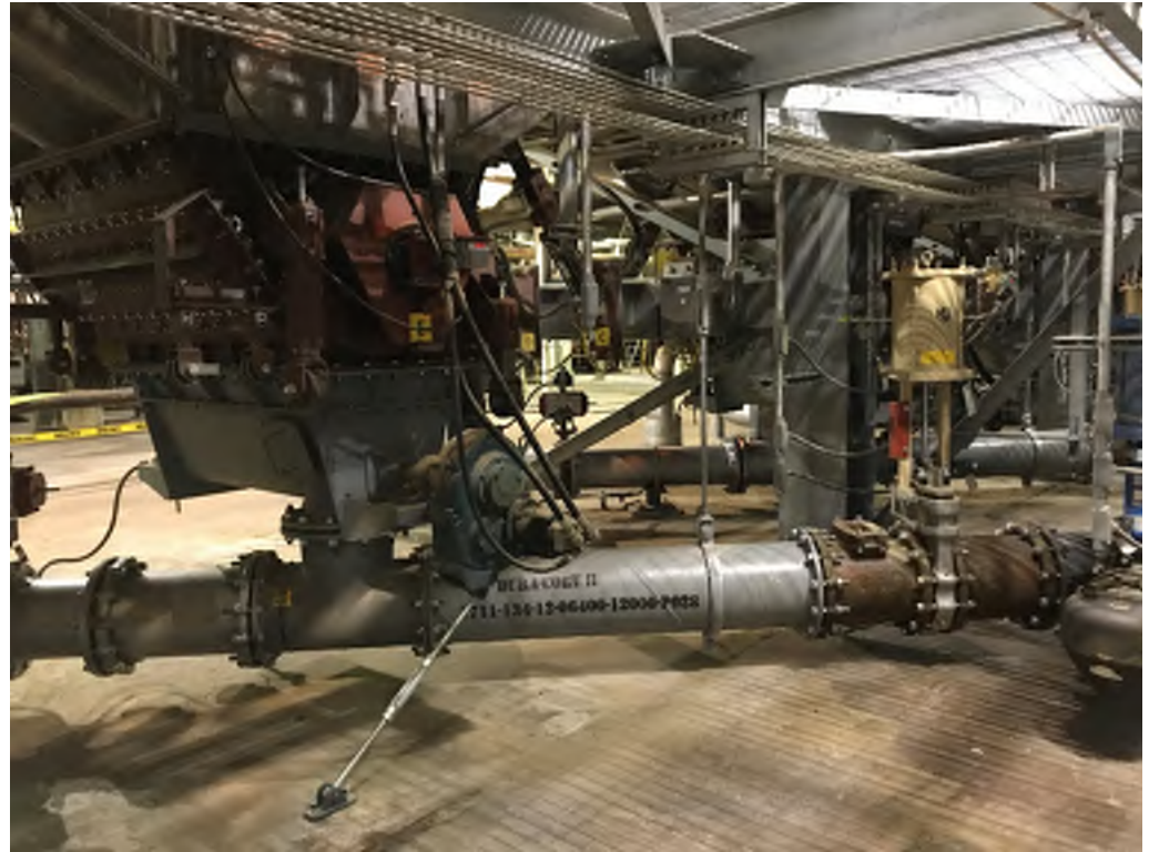
UCC PAX Enclosure and Crusher
